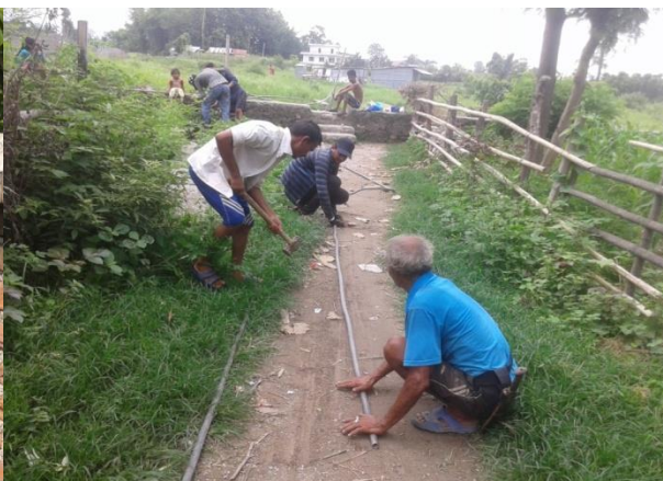
Fixing the water pipeline in Dip School
