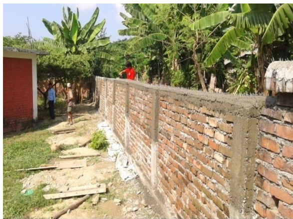
Restored the wall in Dip school collapsed by earthquake
