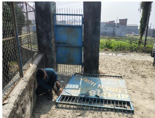
The main gate of home was repaired after the door hinge rusted and broke. The gate has now been fixed for safety purposes, but some painting and minor concrete finishing work are still pending.
